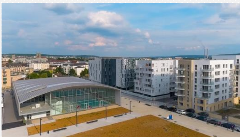
Aquasport, architecte: Marc Mimram
